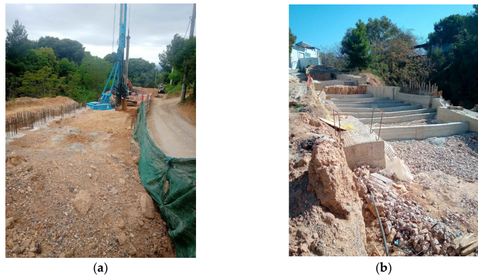
Figure 5. Views from Area A construction: (a) cutter bar machine, (b) pile walls made of intersecting piles (Author's archive).
