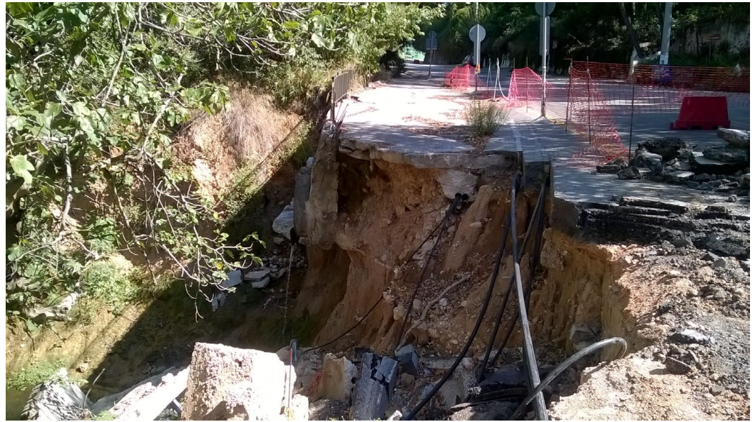
Figure 2. View from one characteristic slope failure (fall) of the examined road (Author's archive).
