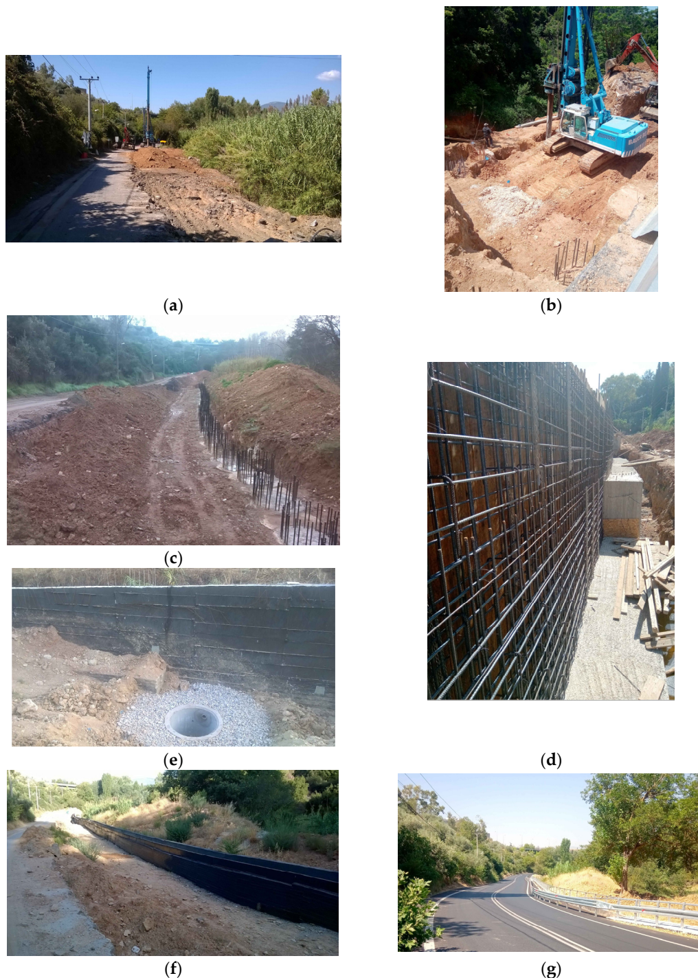
Figure 6. (a–g) Different successive steps of pile wall construction of Areas B to D (Author’s archive). In Figure (e), a view from the drainage system (for lowering the potential pore water pressures and accomplishing adaptation to possible disruption from heavy rainfall episodes) is depicted. Figure (g) is associated with the accomplishment—end of the technical works in September 2023 in the examined segment of the road (Author’s archive).
