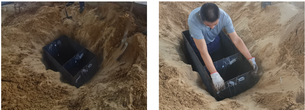
Figure 8. Backfilling of the diaphragm wall installation.
