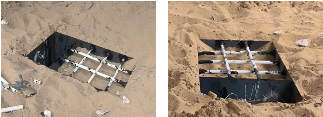
Figure 7. Test excavation process.
