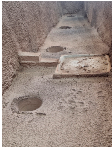
Figure 25. Configuration SP-K4 with the installed impact pad “SPHERC-K4” in the tested tundish.
