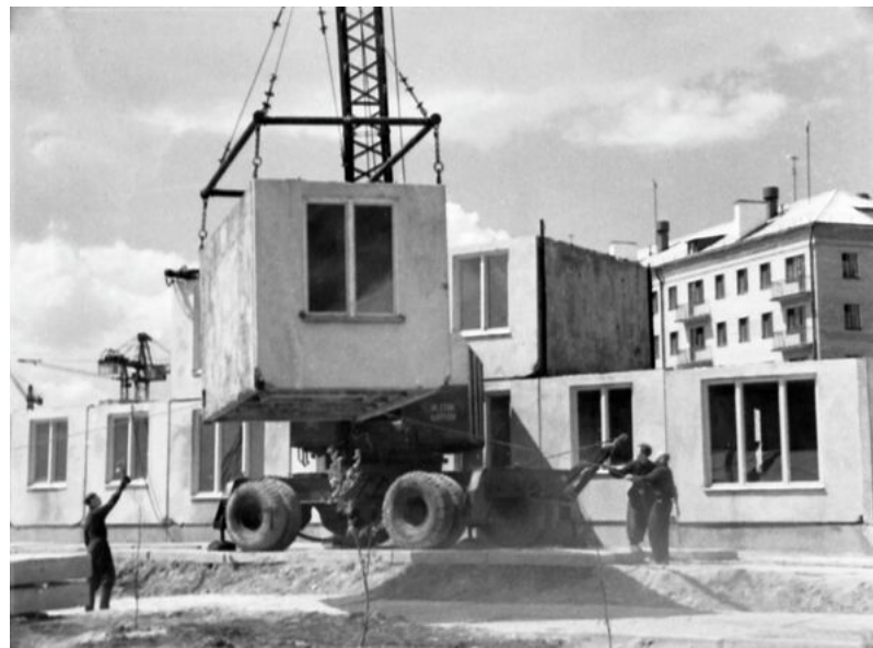
Figure 1. Installation of volumetric blocks.
