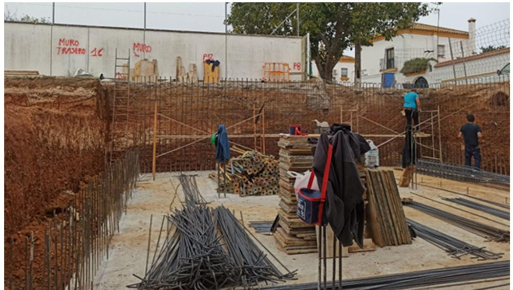
Figure 1. State of the Work in the Initial Phase of Placement of Wall Reinforcements.
