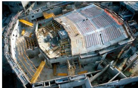
**Figure 2.** Santa Cecilia Hall (Rome): plenum construction phase, with completed diffusers' installation (colored red).
