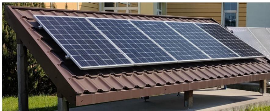
Figure 15. 1.55 kWp research PV installation.
