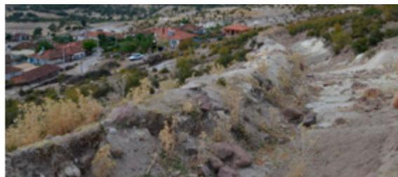
**Figure 4.** Trenches dug to reduce the risk of rockfall; their width reaches 2 m and depths up to 1 m.
