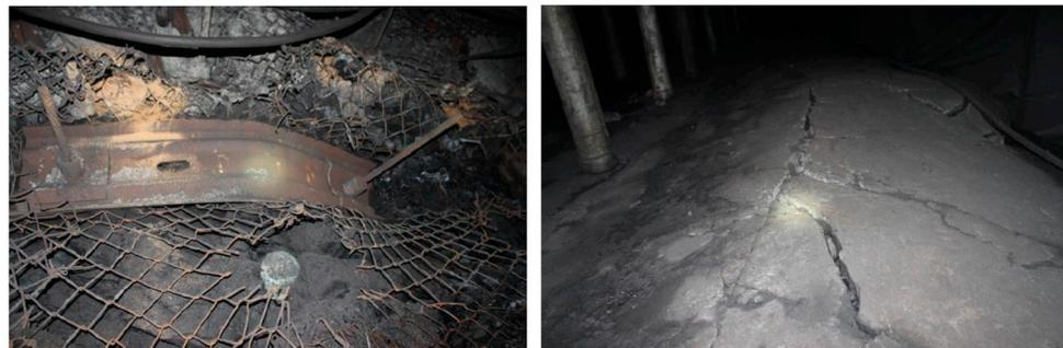
Figure 4. Strong mine pressure behavior of 5204-2 roadway.
