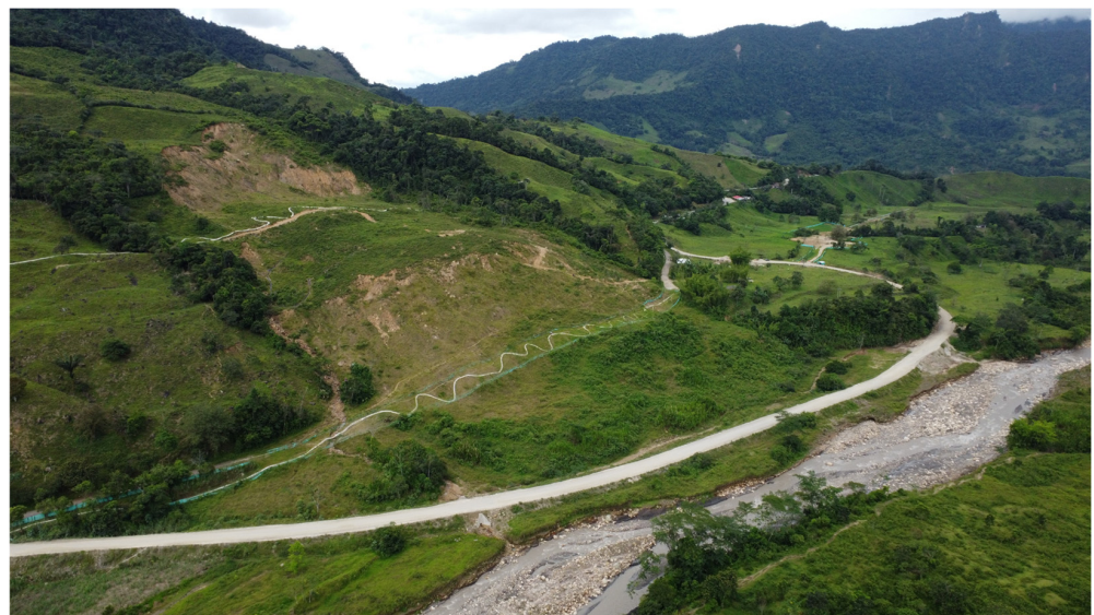
Figure 3. Aerial view of the landslide in 2021.
