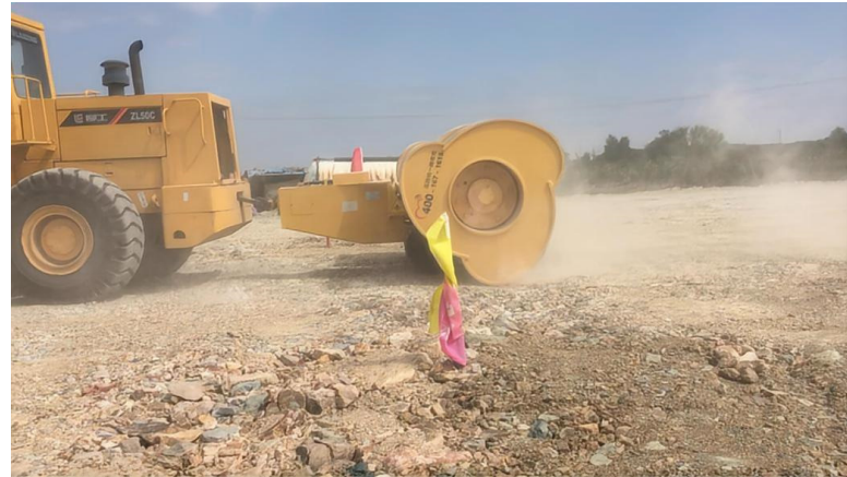
Figure 3. YCT32 16.5-ton three-sided impact roller.
