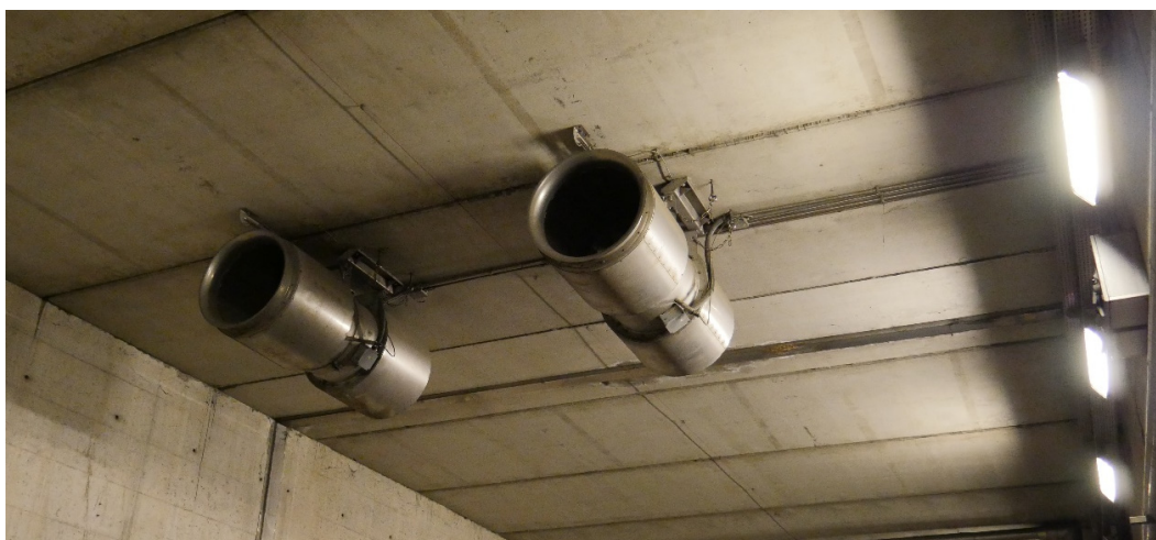
Figure 2. Example of a pair of jet fans anchored to the tunnel roof, used in the longitudinal ventilation of a one-way road tunnel, with airflow in the same direction as the vehicular flow.
