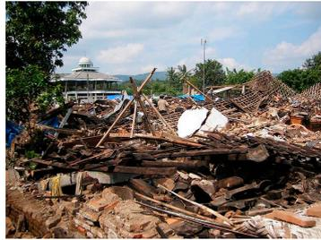
**Figure 4.** Brick masonry damage from Central Java Earthquake (2006).
