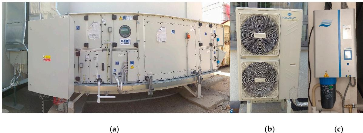
**Figure 4.** Location of HVAC equipment: (a) ventilation unit, (b) heat pump, and (c) air humidifier.
