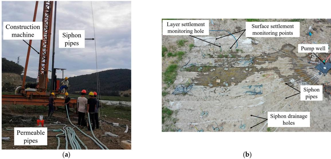
**Figure 10.** The figures of field test. (a) Construction of siphon drainage holes. (b) Top view of field test.
