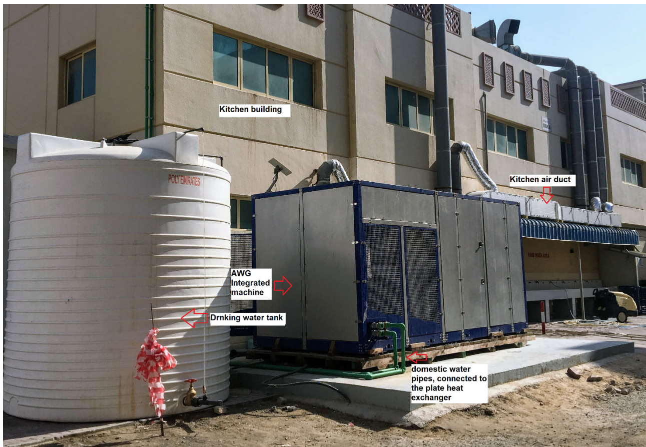
Figure 4. AWG integrated machine installation.
