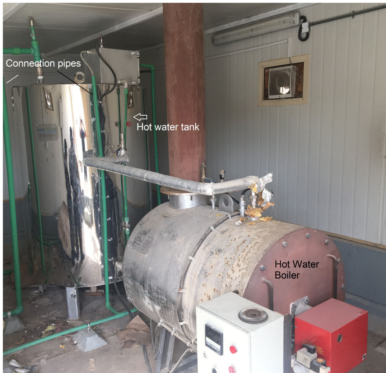
Figure 5. Hot water tank and LPG boiler. In the image, green pipes, connecting the integrated machine to the hot water tank, can be seen.
