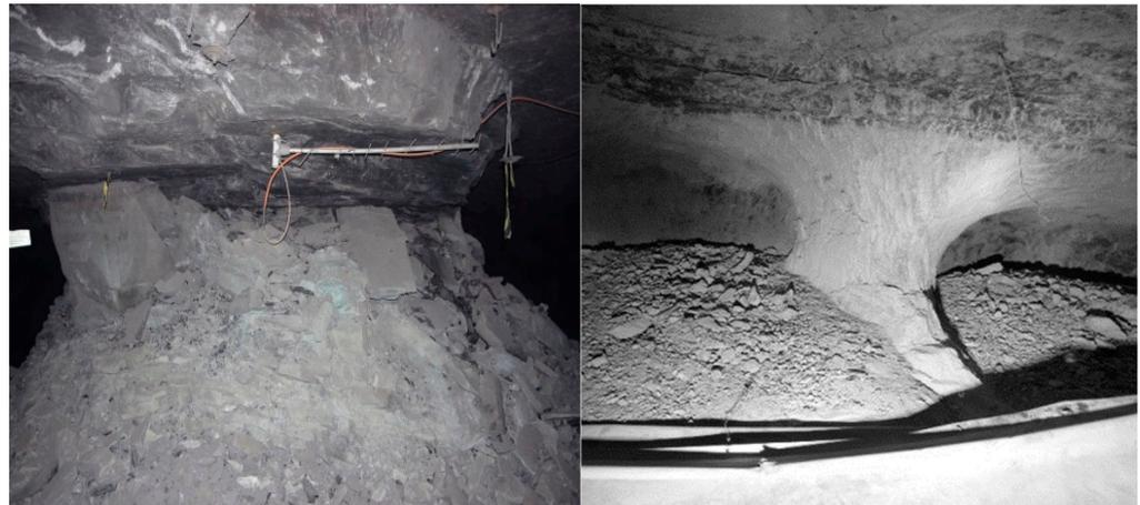
**Figure 5.** Views of damaged mine workings with inclined sidewall surfaces: **(left)**—long pillar at an intersection in Rudna mine, **(right)**—sidewall of a rectangular gallery with inclusion of competent rocks—Polkowice-Sieroszowice mine after blasting works in the close neighborhood, February 2016.
