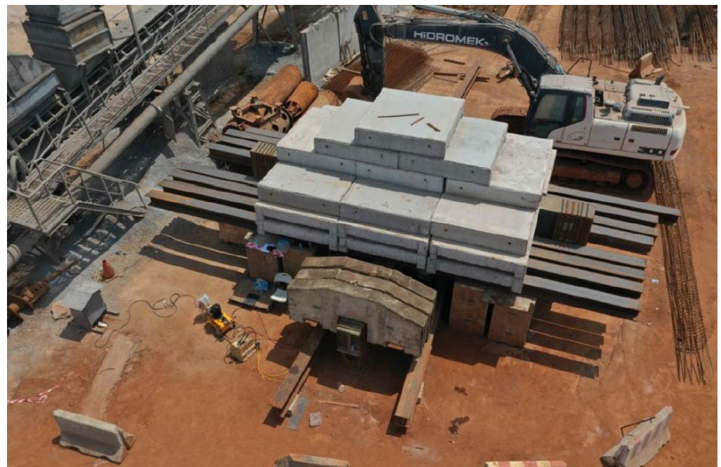
Figure 12. Pile load test set-up.
