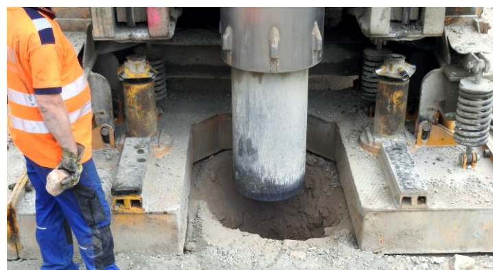
Figure 17. Preliminary hole for pile placement.
