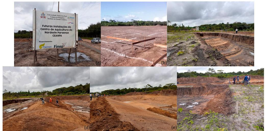
**Figure 9.** Aquaculture operations in Area 1: (a) Installations; (b) Demarcation of the ponds; (c–f) Excavated ponds.
