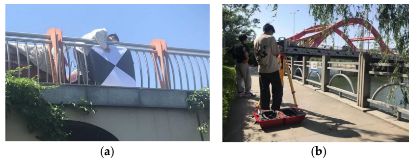
Figure 6. Test site. (a) Layout of deformation point beacons; (b) overview of five warp point beacons.
