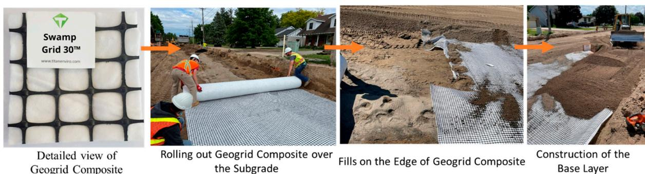
**Figure 2.** Installation of geogrid composite on the subgrade.
