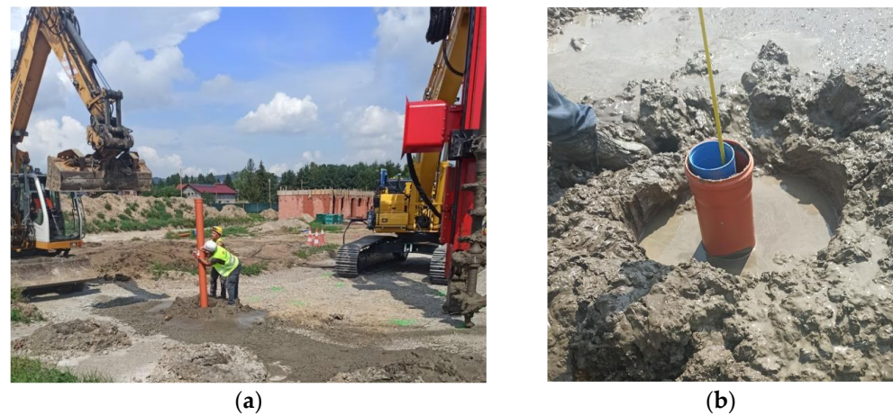
Figure 4. “Pipe in pipe” probing system. (a) Installation of the pipe in the “fresh” column. (b) Pipe head just after its plunging.
