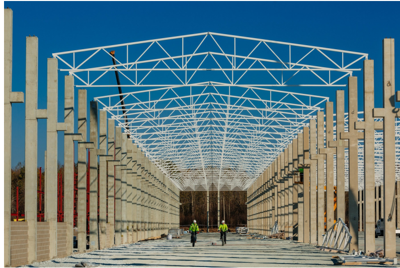
Figure 3. Construction of a hall with a truss system [26].
