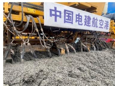
(b) Vibratory liquefaction of concrete
