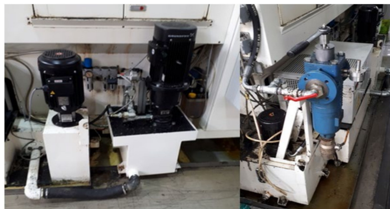
Figure 5. Standard cooling pump, high pressure pump, and Mahle filter unit.
