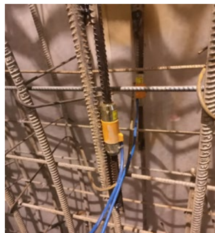
Figure 5. Smart string-type steel stress meter.
