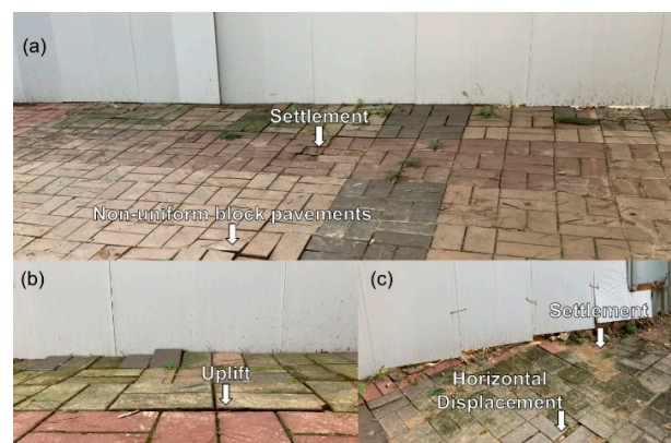
Figure 1. Displacements of paving blocks adjacent to the deep excavation site: (a) settlement and non-uniform block pavements; (b) uplift; and (c) settlement and horizontal displacement.
