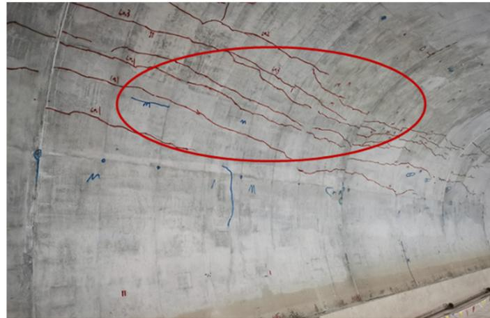
Figure 6. Photograph of longitudinal cracks on the right arch waist.
