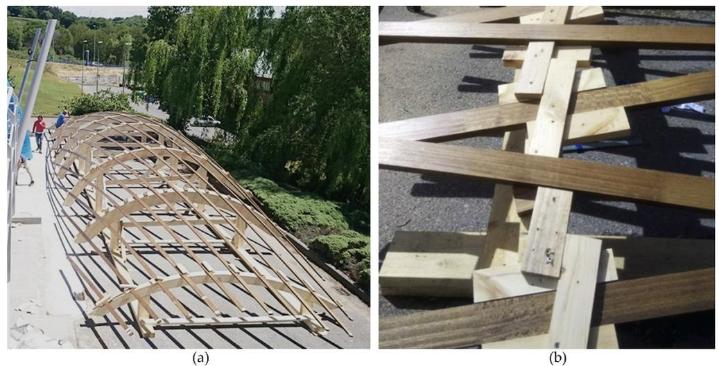
**Figure 26.** Gridshell during construction: (a) Curving process of the first family of laths; (b) Detail of the placement of the laths on the formwork.
