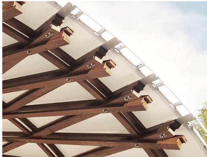
**Figure 27.** Detail of the end of the laths at the short edge of the structure.
