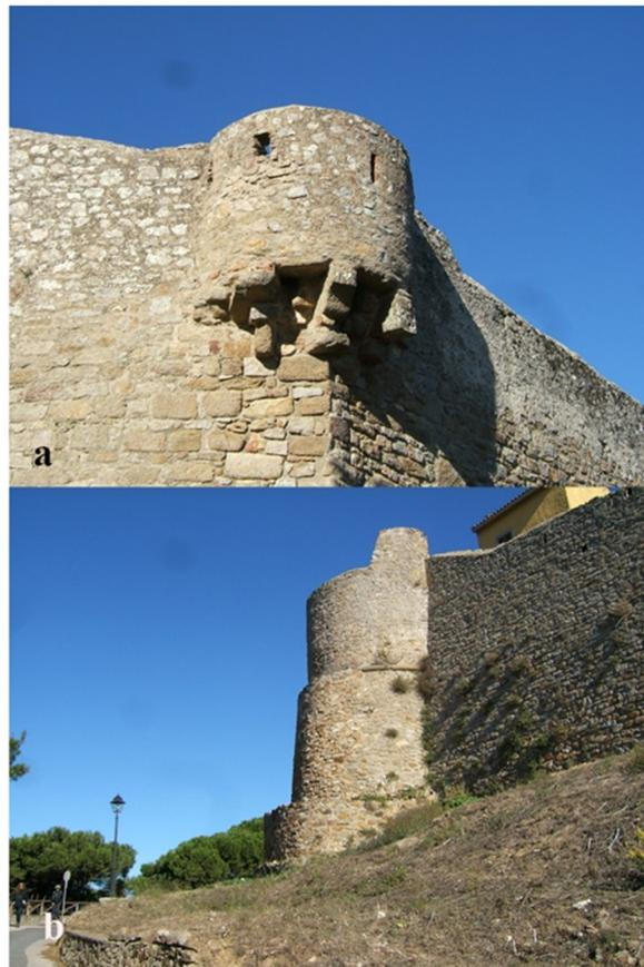
**Figure 3.** Giglio Castello: walls of the 16th century, built with granite ashlars (a). Giglio Castello: detail of a tower of the city walls resting on a granite outcrop (b).
