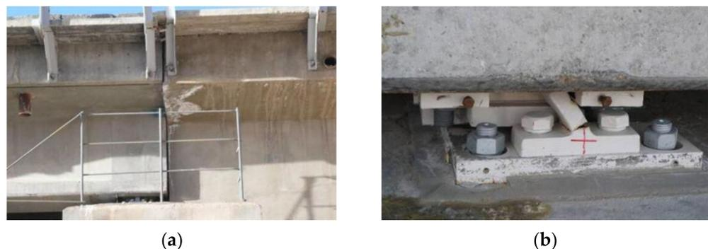
**Figure 2.** Bridge damage of Qinghai–Tibet railway. (a) Direct contact of adjacent beams. (b) Fracture of bearing limit block.
