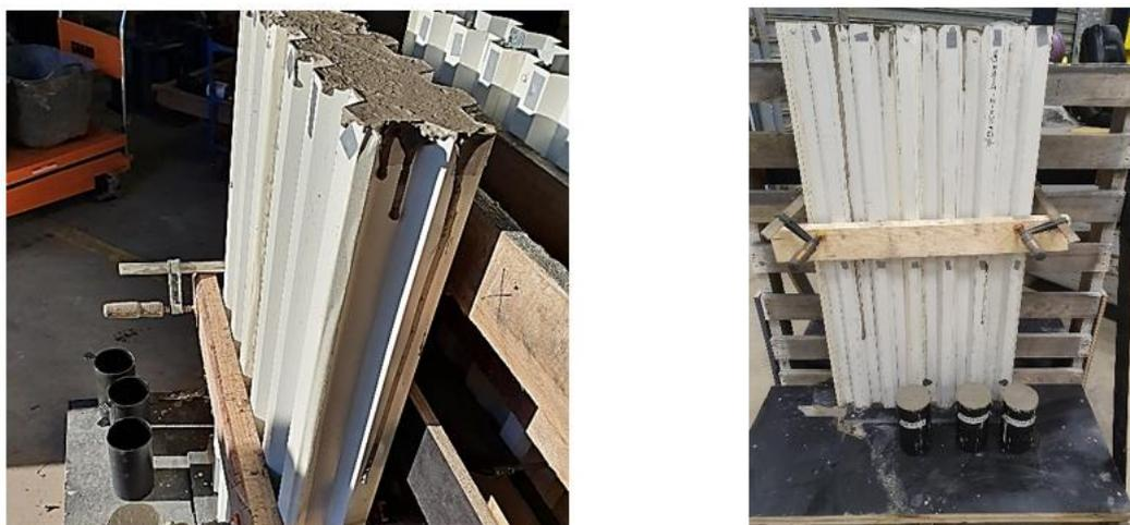
Figure 3. Casting of panels.
