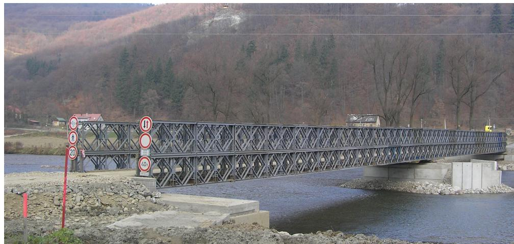
**Figure 2.** Bailey bridge (TD-36 + 36) placed on construction site road over Orava river (Slovakia).
