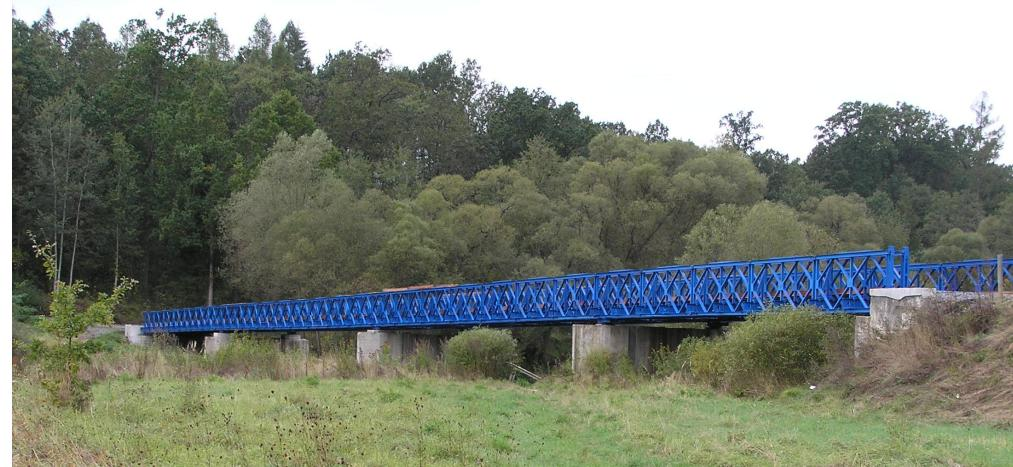
**Figure 3.** ‘Long-term’ temporary bridge Bailey bridge (DS-15 + 21 + 27 + 21) over Lužnice river (Czech Republic).
