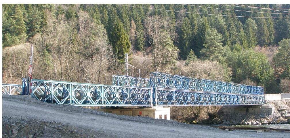
**Figure 1.** Bailey bridge (TS-12 + TD-33) over Vah river during construction (Slovakia).
