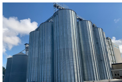
Figure 2. View of silos battery used for grain storage with capacity of 3955 tons (Campo San Martino, Italy).
