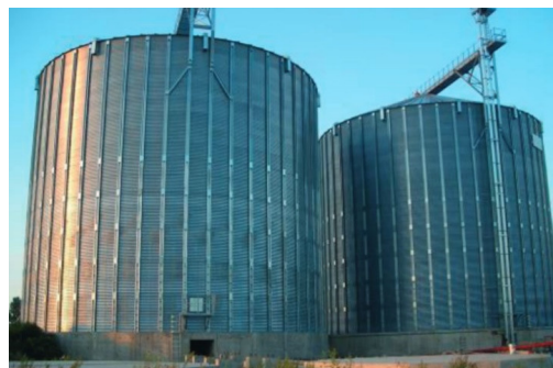
Figure 5. Silo corrugated walls in combination with the vertical stiffeners (well-known as silo columns). Source: [79].
