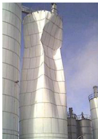
Figure 7. Extreme damage in grain silo caused by asymmetric flow pattern. Source: [29].
