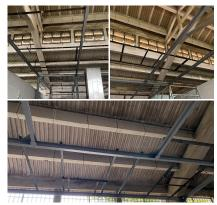
(a) The ceiling space at BK-RECME before in- (b) Steel beam frame installed on the ceiling stalling the system
