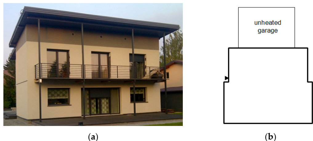
Figure 6. Photographs of the analyzed building: (a) south facade of the analyzed single-family building with an additional self-supporting light balcony system made of steel profiles; (b) layout of the analyzed building.
