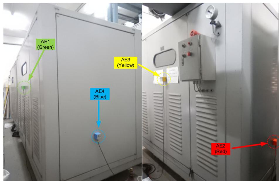
**Figure 4.** Installation of Acoustic Emission Sensor (AE1–AE4) with housing of transformer.
