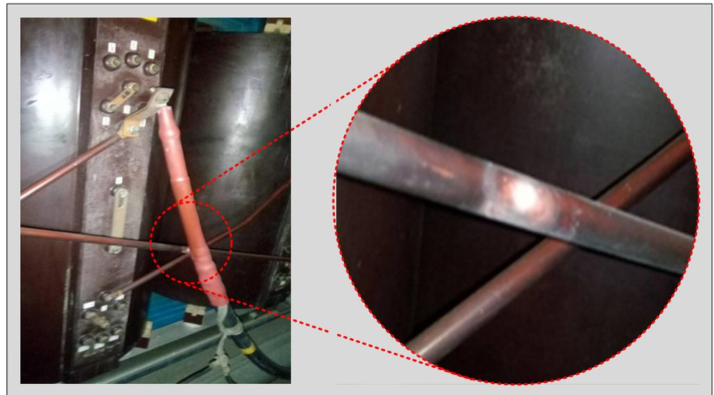
**Figure 15.** The evident of partial discharge on the insulator surface of high voltage side.
