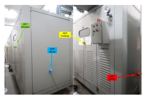
Figure 4. Installation of Acoustic Emission Sensor (AE1-AE4) with housing of transformer.
