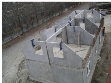
**Figure 22.** Mounting the attic (Photo archive: Kalús, D.) [13].
