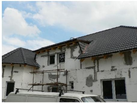
**Figure 24.** View of the implementation of the insulation of the perimeter panels. (Photo archive: Kalús, D.) [13].
