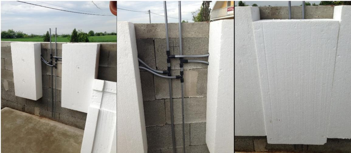
**Figure 15.** The principle of the contact thermal insulation system with ATP. [Author: Kalús].
