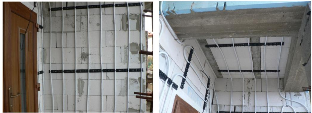
**Figure 27.** Placing pipes of active thermal protection on the facade. [Author: Kalús].
