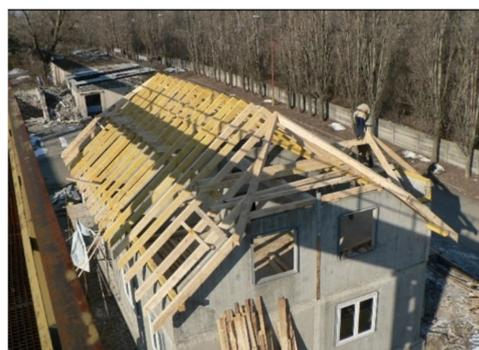
**Figure 23.** View of the realization of the wooden truss. (Photo archive: Kalús, D.) [13].
