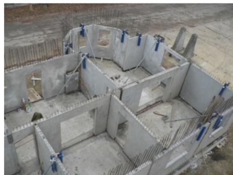
**Figure 21.** Completion of the ground floor assembly. (Photo archive: Kalús, D.) [13].
