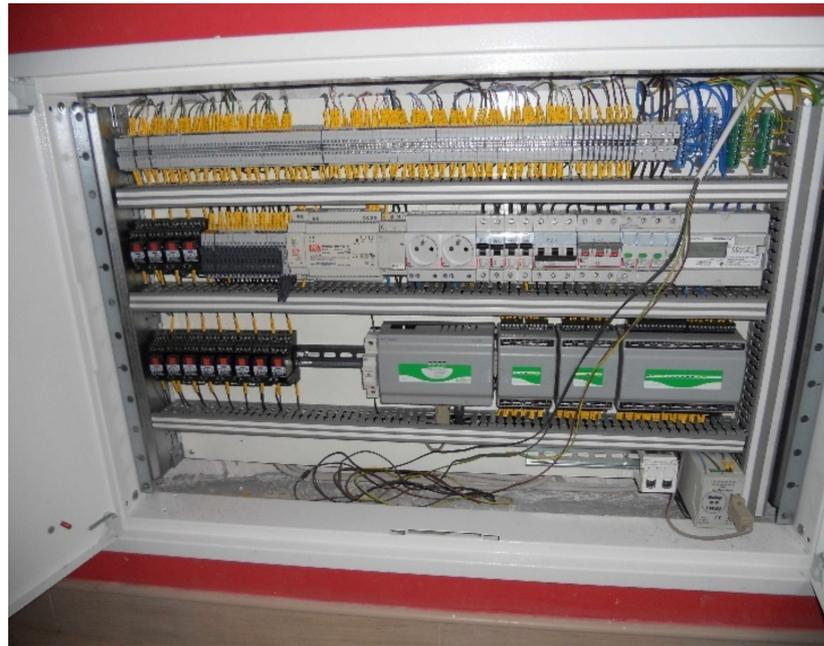
Figure 3. Measuring and recording control panel installed in the experimental house EB2020 [15,16].
