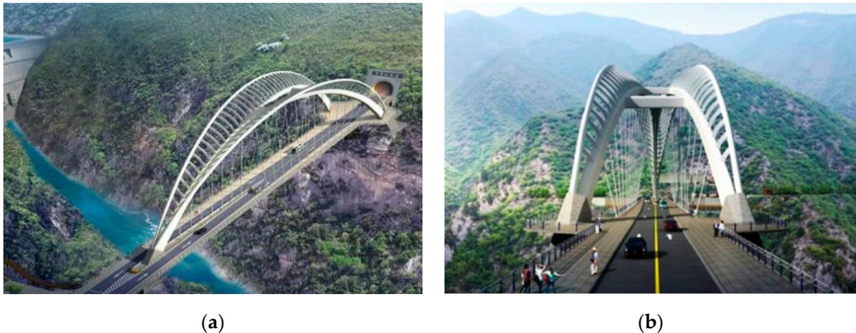
**Figure 1.** Three-dimensional rendering of main and secondary arch collaborative Y-shaped steel box arch bridge: (a) isometric drawing; (b) side-view drawing.
