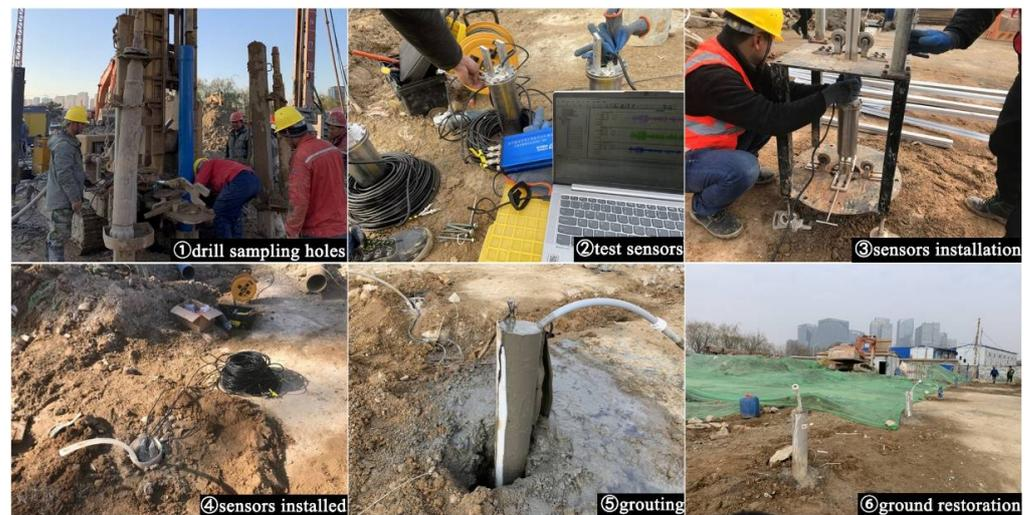
**Figure 6.** Installation process of the sensors.
