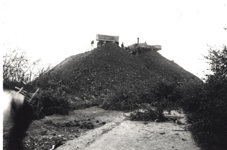
Figure 2. Image showing end-tipping construction method, used during early construction of the British railway, at Blackbird Road, Leicester circa 1897 (Photo reproduced with permission of Record Office for Leicestershire, Leicester and Rutland).
