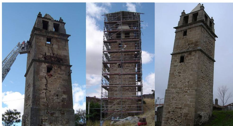
Figure 7. Overview of the Mogadouro tower before, during and after the rehabilitation works.
