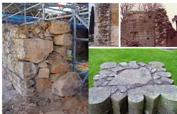
**Figure 1.** Examples of ancient masonry section with complex arrangements of units.
