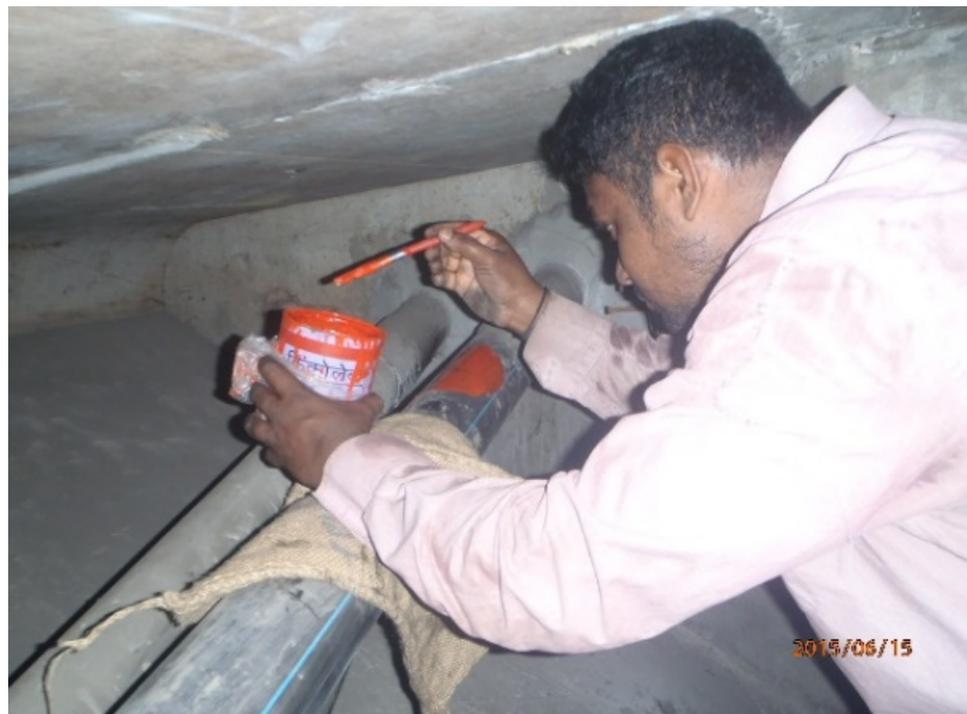
**Figure 14.** Marking suspect locations along post-tensioning elements.
