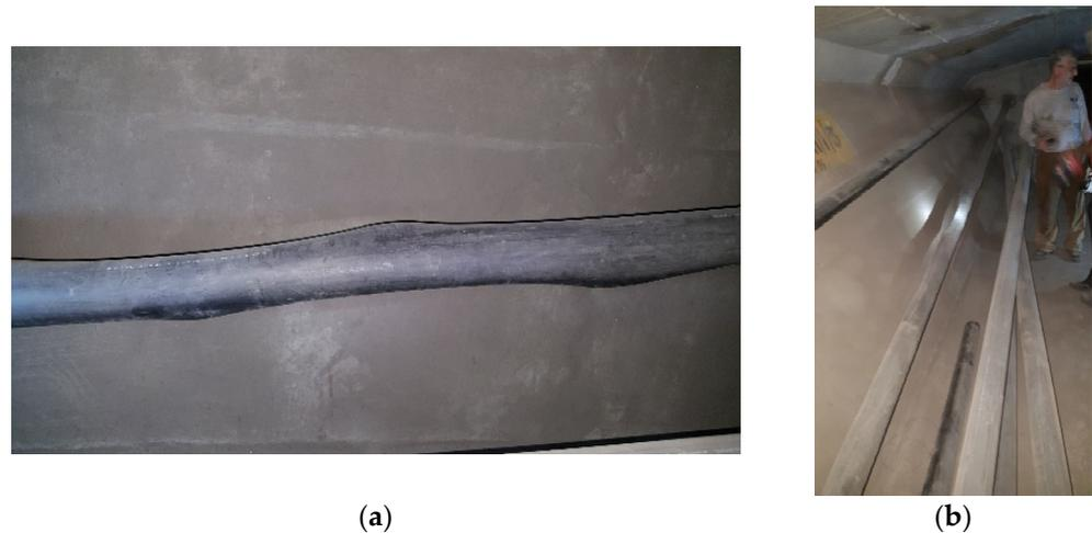
**Figure 13.** Spot inspection activities (case study) to verify the current condition of the bridge; (a) one of defected external tendons, (b) inspectors during spot inspection.
