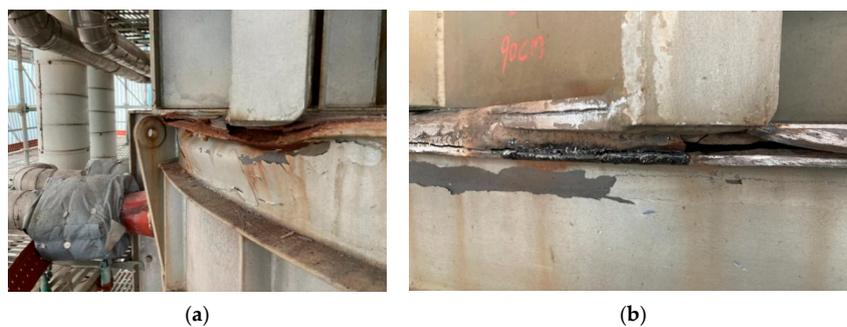
Figure 6. Fatigue failure of the support frame before reinforcement: (a) at the south-east side; (b) at the north-west side.
