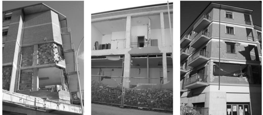
**Figure 1.** Partial and complete out-of-plane collapses of infilled walls during the L'Aquila earthquake (2009), Italy.
