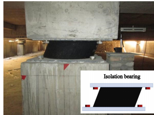
Figure 14. Distorted isolation bearing.
