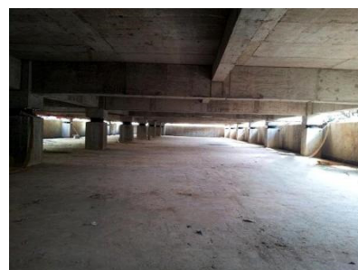
Figure 4. Isolation overhaul layer.
