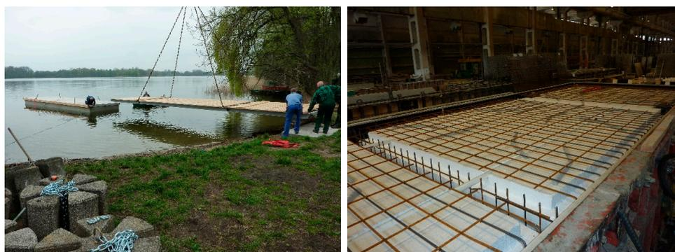
**Figure 9.** The pontoon during execution with visible reinforcement and a partition in the centre (left) and during launching (right).
