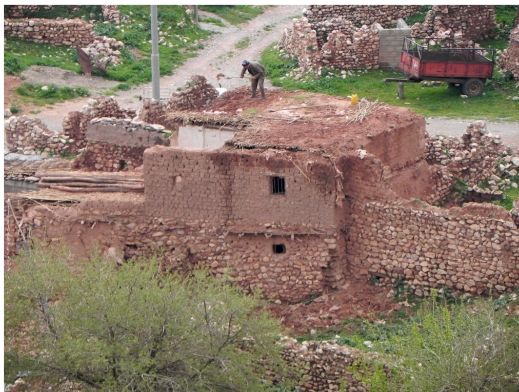
Figure 11. Photograph from field research capturing the dismantling of older buildings in the inner part of the city to obtain a key building material: timber (author: Karel Nováček).
